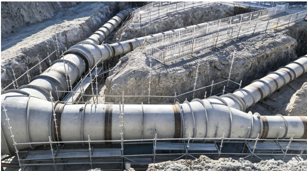
XINJIANG ZD WATER SUPPLY PROJECT (PHASE II)
